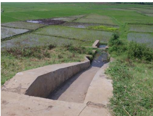
The spillway seemed to be too small compare to the reservoir of the dam.
