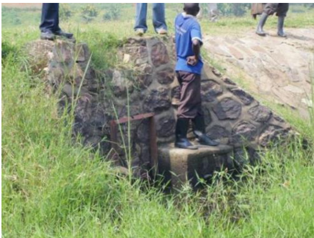
The spillway seemed to be too small compare to the reservoir of the dam.
