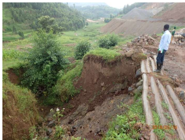
(Figure17: Erosion control is very important)
