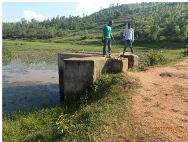
(Figure15: Check the Dam)
